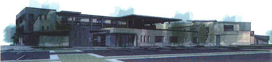
view from south-west
